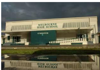
Mel-Hi's 52 year old gym will be torn down this spring giving way to a $10.5 million facility.
